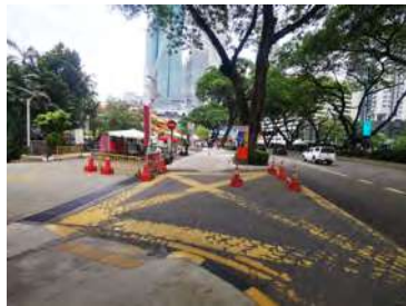
Absence of appropriate crossing marking and apparatus (e.g. pedestrian crossing signage)
