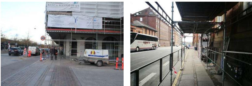
Photo 4.3: Cover over walkway at construction site in Copenhagen, Denmark
