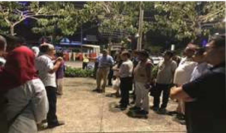
23 Julai 2018 : Lawatan Delegasi Infrastructure Citynet & KLRTC XXXII ke Tapak Projek River Of Life, Precinct 7
