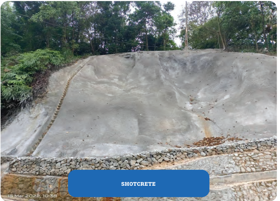
SHOTCRETE WITH SOIL NAILING
